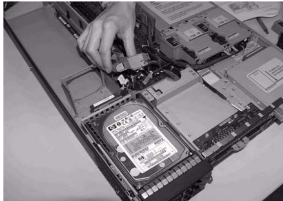
Figure 8-11 Lifting the Fan Power Bridge
